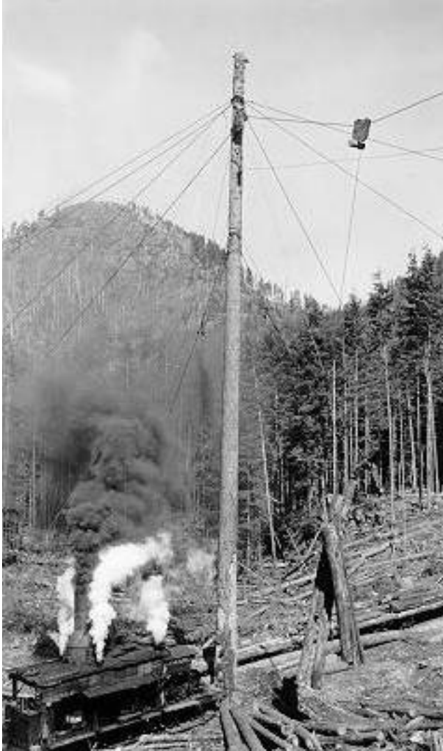
Figure 3: A yarder using a skyline to bring logs to the landing. MacMillan Bloedel Limited fonds; BC 1930/19/50; date listed as 1942.
