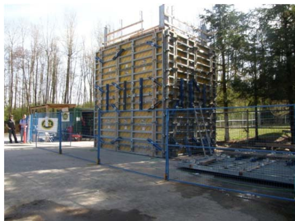
Figure 29 Construction of indoor-to-outdoor sound transmission suite
