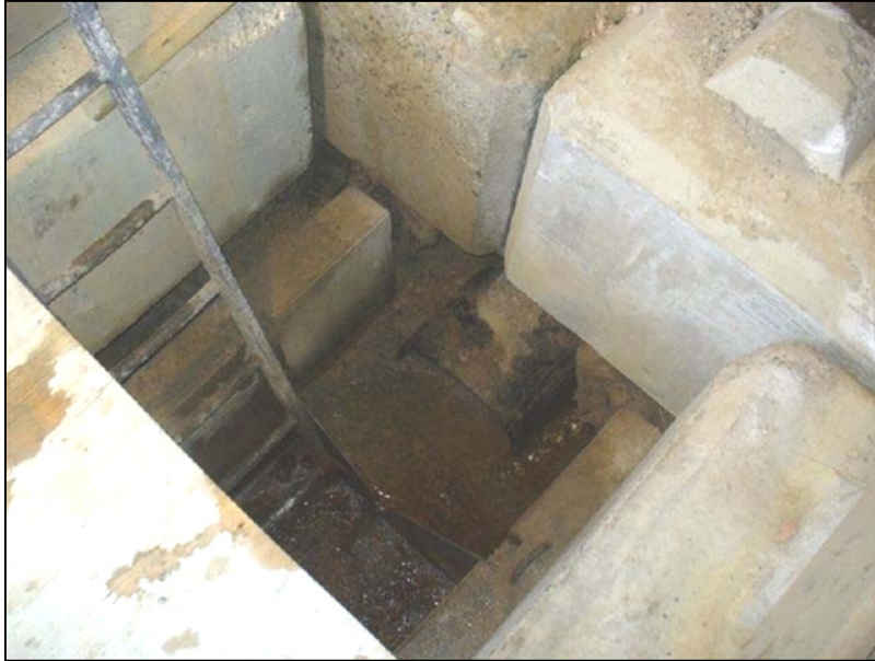
Figure 3-8. The sump at the bottom of the sampling shed. Note the weir to the bottom-right of the ladder (Courtesy of WorkSafeBC).
