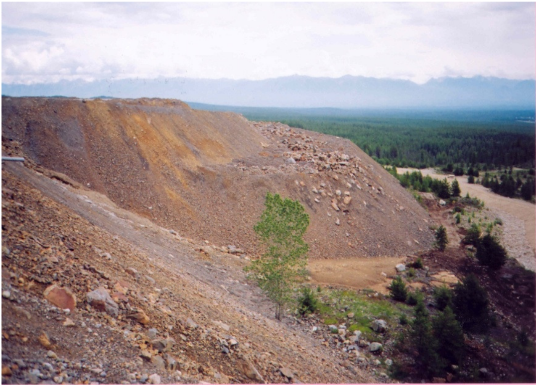
Figure 3-1. No. 1 Shaft Waste Dump at the Sullivan Mine prior to regrading and covering with glacial till (Reports of the Technical Advisory Committee of the Sullivan Mine accident, 2007, by permission Teck Metals Ltd).
