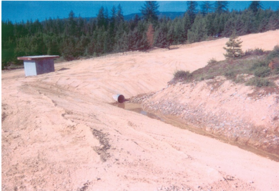
Figure 3-2. Seepage collection ditch in September 2005 prior to covering with glacial till (Phillip et al., 2008, by permission).
