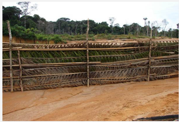
4 – Tailings containment with barriers of Palm trees
