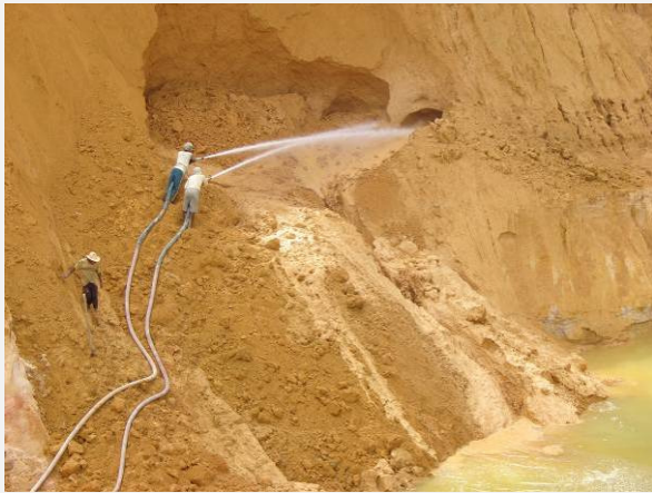
1 – Use of hydraulic monitors for excavation
