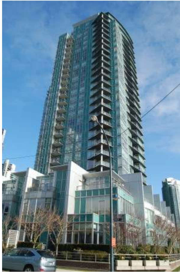
Figure 3: The “tower-podium” is a commonly used building typology in False Creek North used to accommodate density while maintaining a “friendly face” to the street. Here, townhomes are used in the podium.
