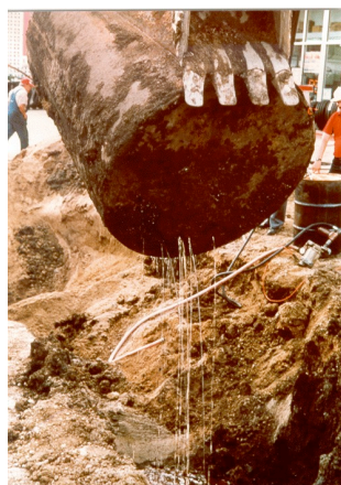
Figure 9: Removing a leaking underground tank
