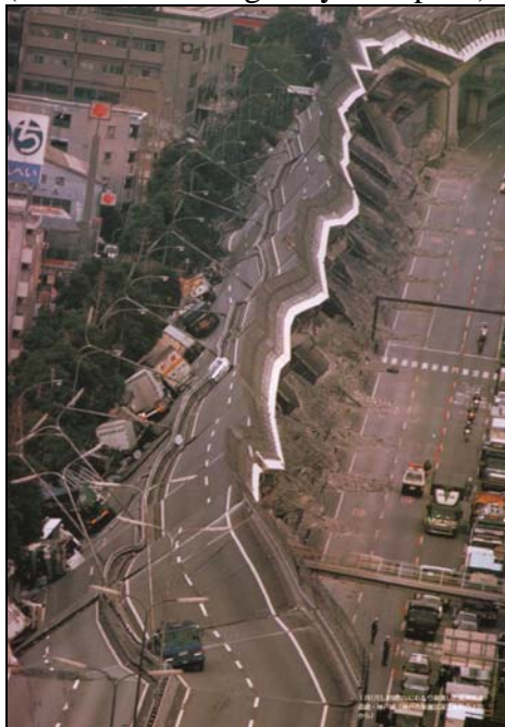
Figure 4 3: Hanshin Highway (600 meters of highway collapsed)
