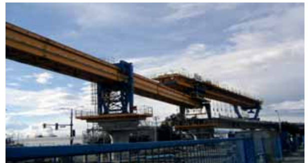
Photo 8. Segments post-tensioning underway 2
