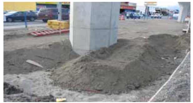
Photo 6. Backfilling underway
