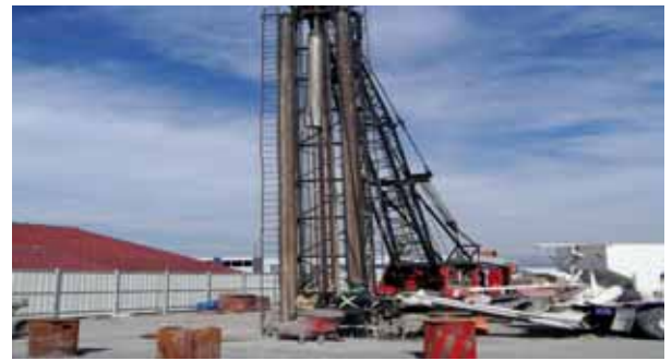
Photo 2. Drilling of piles
