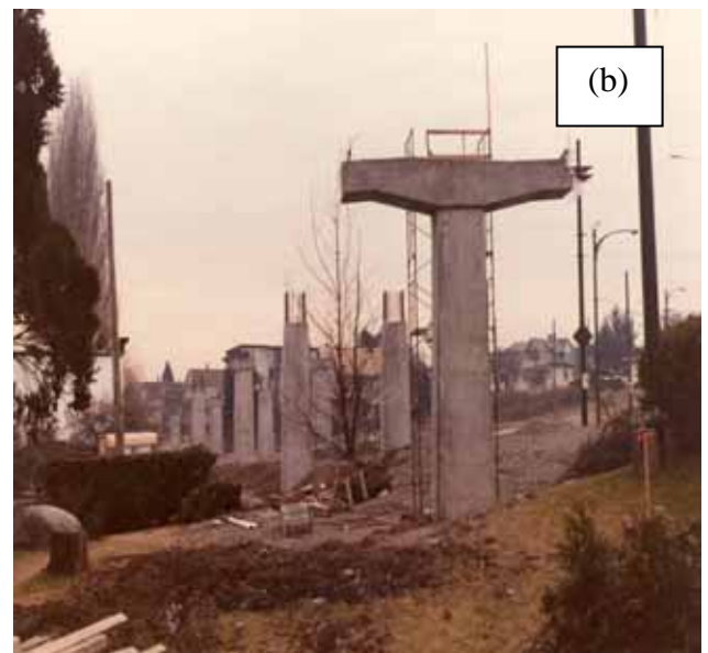
Figure 1.2 Process view – (a) Scoping of project activities by construction phase; (b) Photo of completed fixed and expansion columns; (c) Activity/production data specifying locations worked, production rate and activity type; (d) Planned & actual start & finish dates of activity survey and layout.
