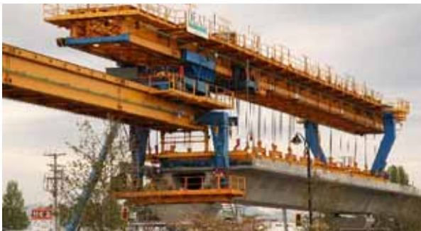
Photo 7. Segments installation is in progress 2
