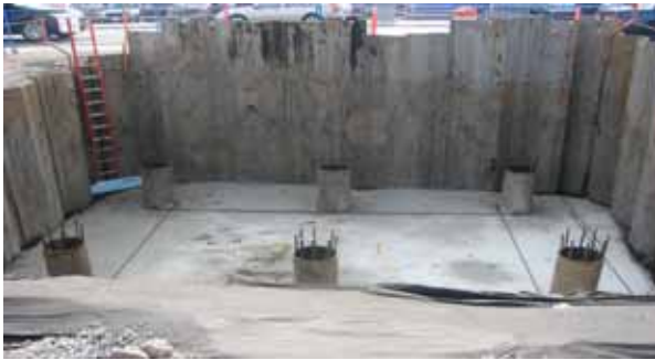
Photo 3. Pile cap footing poured
