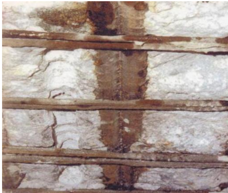
Figure 2.1 Steel reinforcement corrosion in the concrete (Broomfield, 1997)
