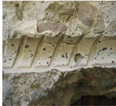
b) Concrete below steel bar (bottom cover)
