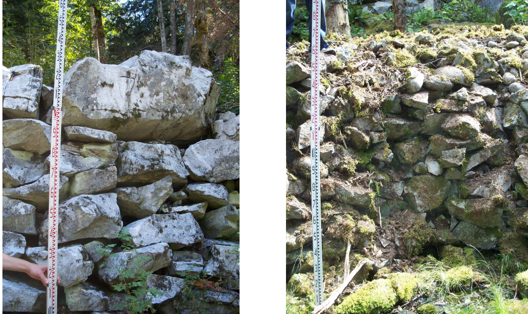
Figure 4.7. Coursed rock features with medium-loose stacking (left) and tight stacking (right).
