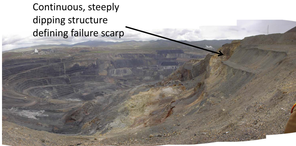
Figure 5.42: Photograph roughly perpendicular to failure slope showing presence of a steep, continuous structure
