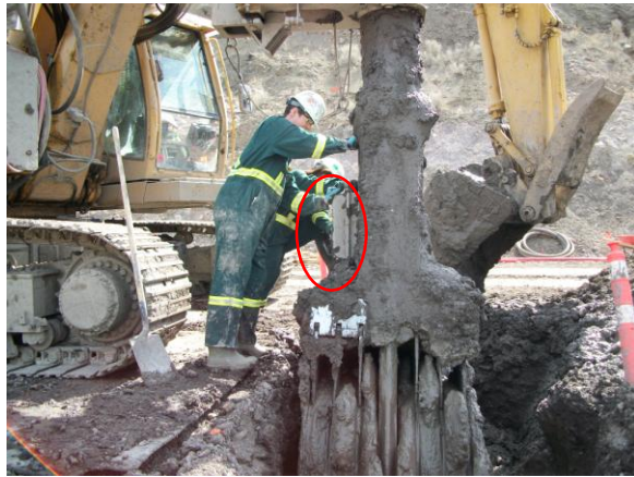
a) Mounting of the Sampler Box
