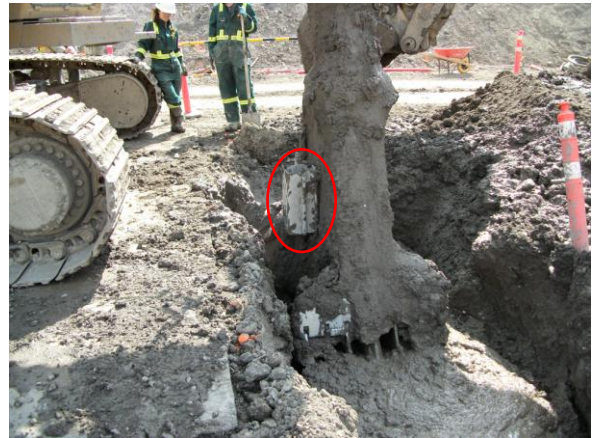
b) Insertion of Sampler Box
