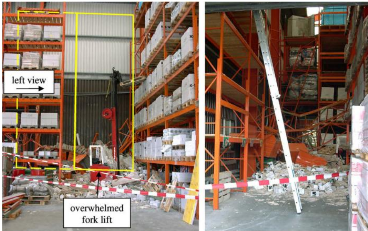
Figure 2.3: Scene of the accident (left: front view with the original position of the rack indicated by yellow rectangles, right: side view) adopted from Affolter et al. (2009)
