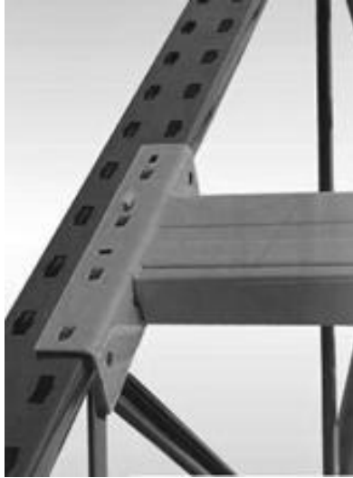
Figure 2.2: A typical RCB beam column joint (adapted from Saar Lagertechnik GmbH (2010))
