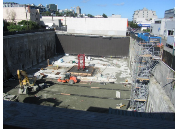
Figure 2.13. Project site after putting grounding wires and reinforcing crane 1 foundation slab
