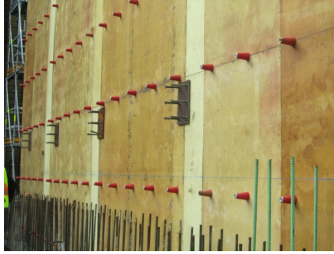
Figure 2.27. Steel embeds installed on the form ready for concrete to be poured
