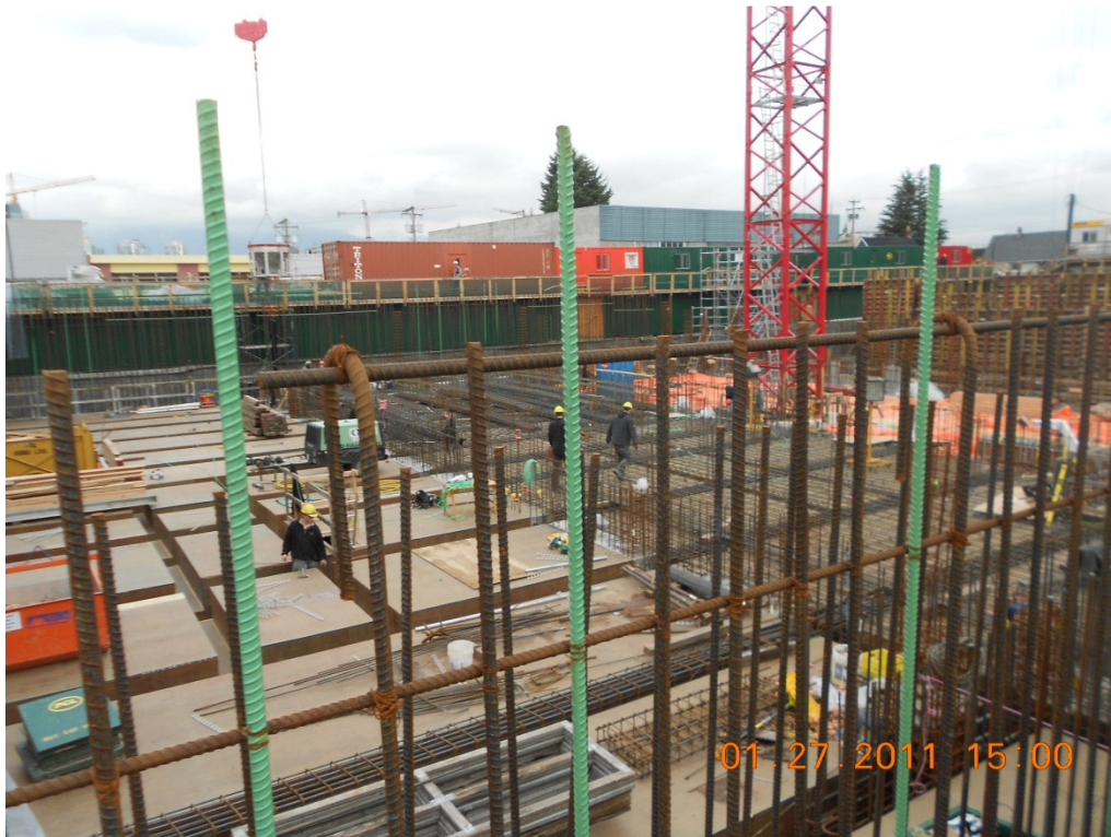
Figure 2.39. Forming the suspended slab on site
