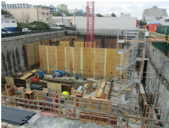
Figure 2.16. Wood panels for forming the walls
