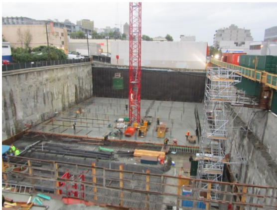
Figure 2.14. Finishing half of foundation slab and reinforcing the other half
