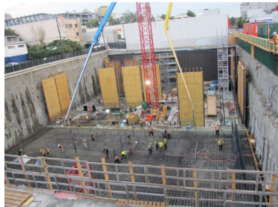
Figure 2.15. Concrete pouring the other half of foundation slab
