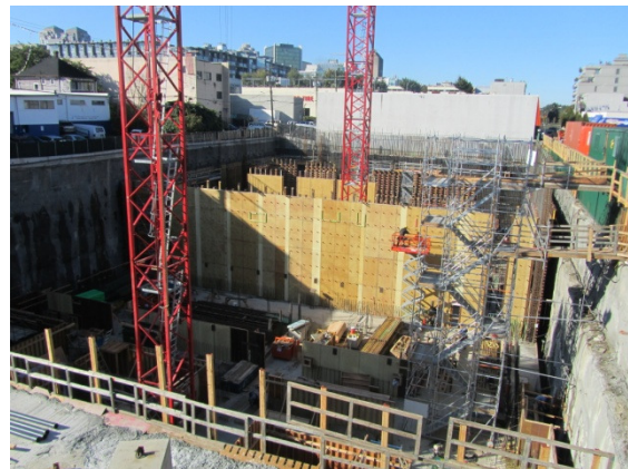
Figure 2.17. Formwork for the west side of the wall along grid line 4 with embeds and location of the ducts on it
