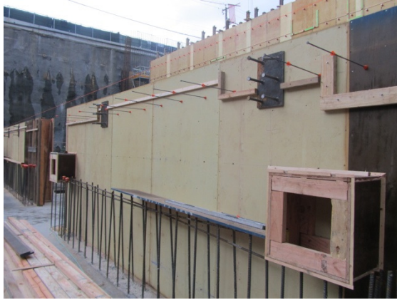
Figure 2.18. Part of a formwork for a wall with the embeds and block-outs
