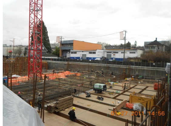
Figure 2.19. Forming suspended slab
