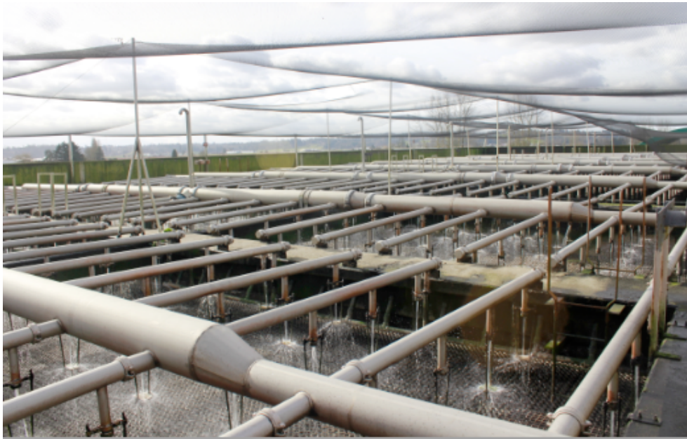
Figure 2.6 Top view of the Trickling Biological Filter
