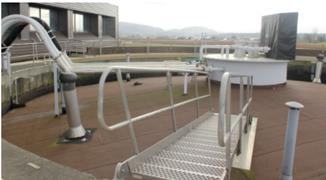
Figure 2.11 Roof of anaerobic digester
