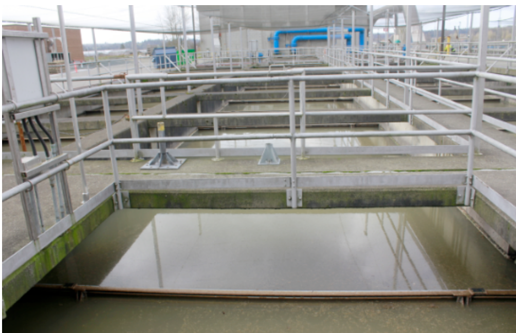
Figure 2.3 Primary sedimentation tank of J.A.M.E.S. WWTP
