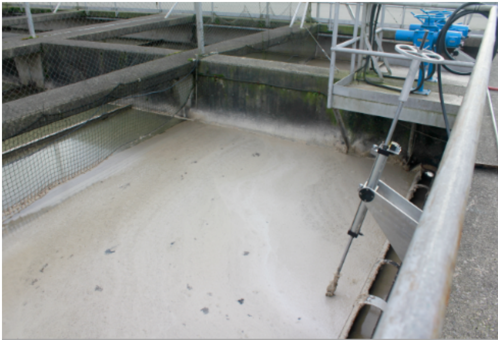
Figure 2.5 Skimming removal tanks of J.A.M.E.S. WWTP
