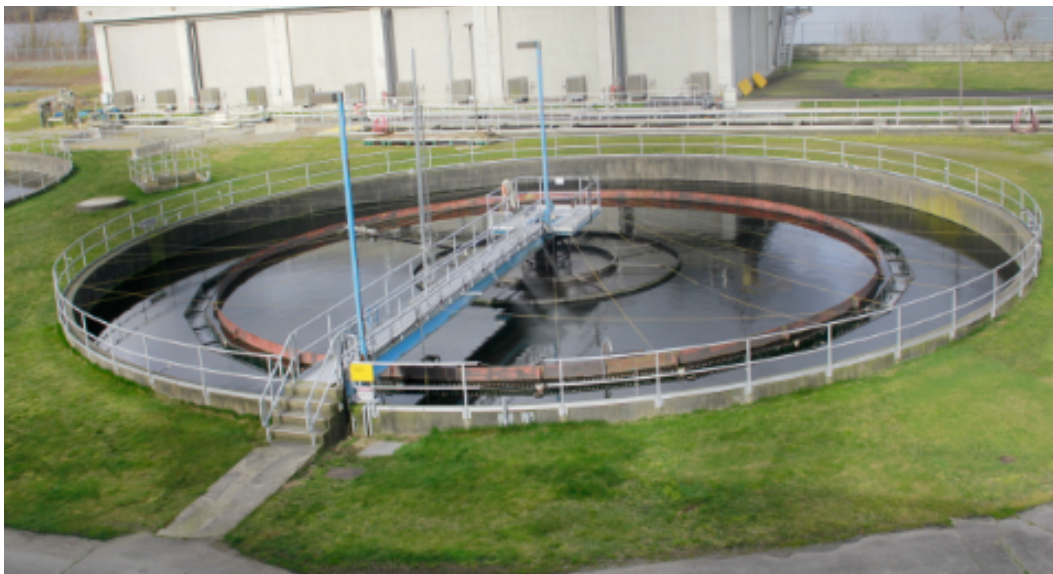
Figure 2.9 Full view of secondary clarifier
