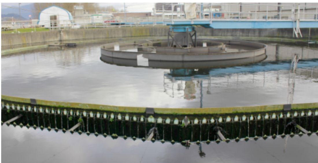
Figure 2.10 Close view of secondary clarifier
