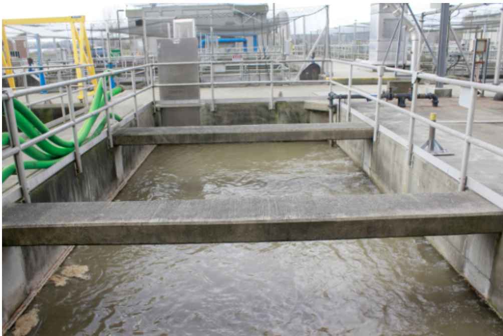
Figure 2.2 Primary grit separation tank of J.A.M.E.S. WWTP
