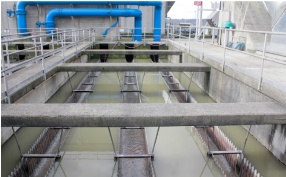
Figure 2.4 Decant of primary sedimentation tank of J.A.M.E.S. WWTP
