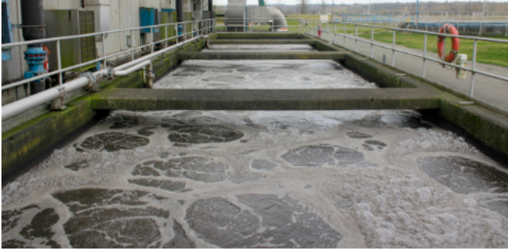
Figure 2.8 Solids contact tank
