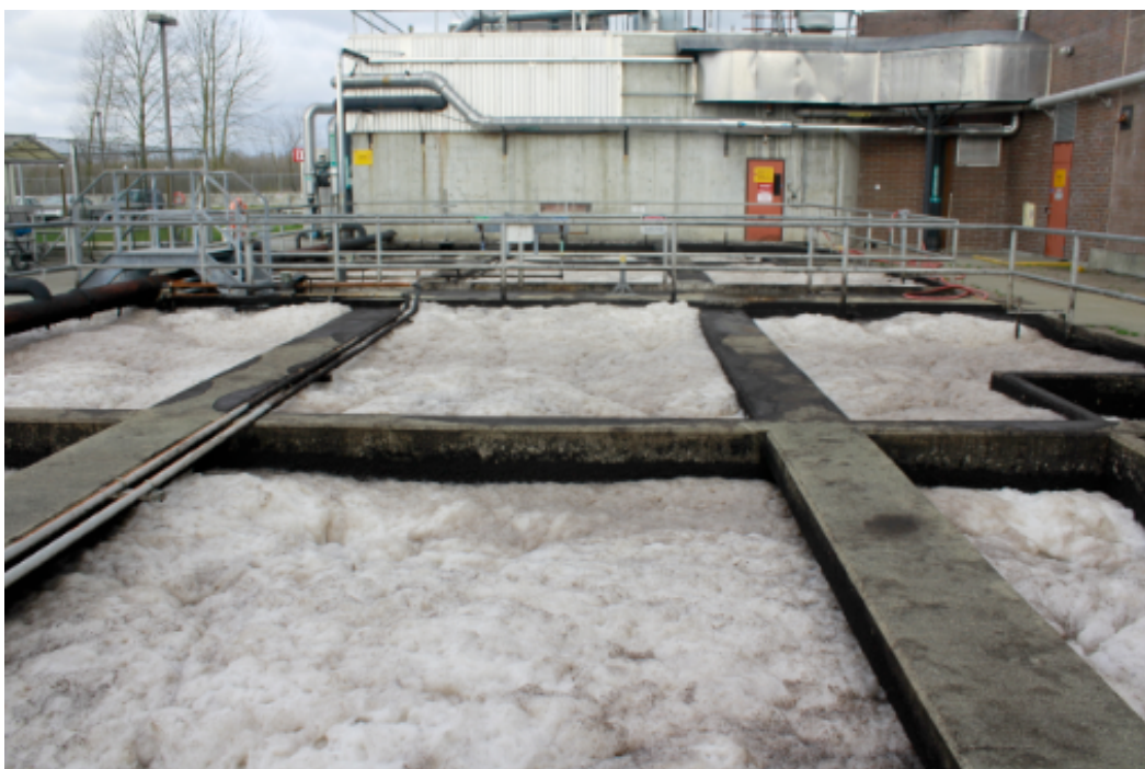
Figure 2.14 Nitrification tanks
