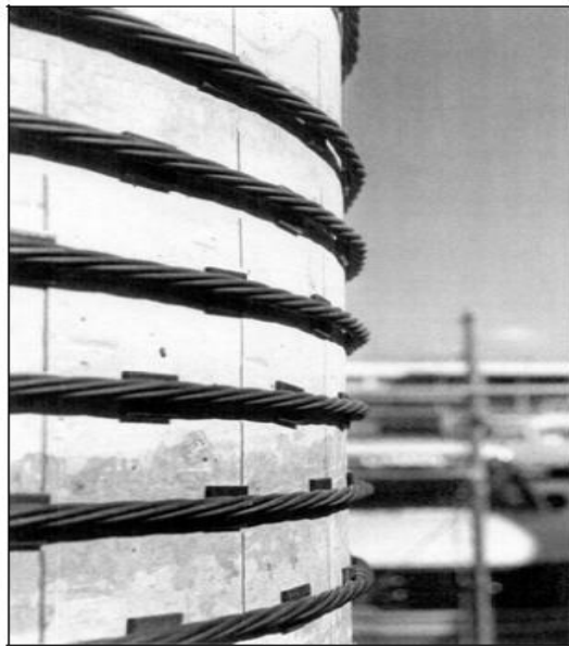
Figure 2.5: Column retrofitting using external prestressing (FHWA-HRT-06-032, 2006)
