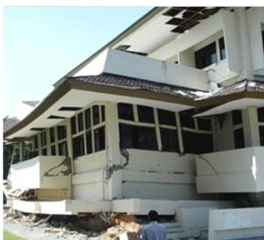
(a) Building collapse due to soft storey effect
