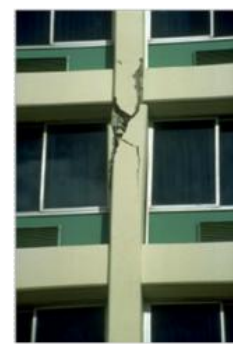
(b) Shear collapse
