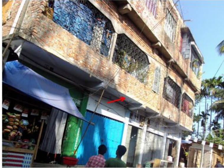
Figure 2-5: Typical heavy overhangs found in Bangladesh
