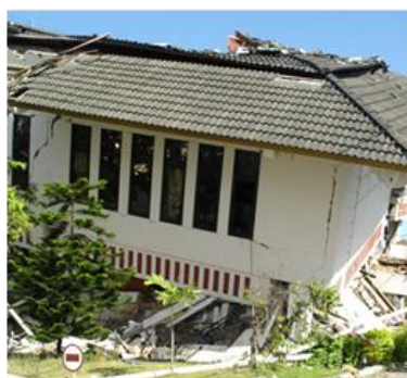
(a) Building collapse due to soft storey effect
