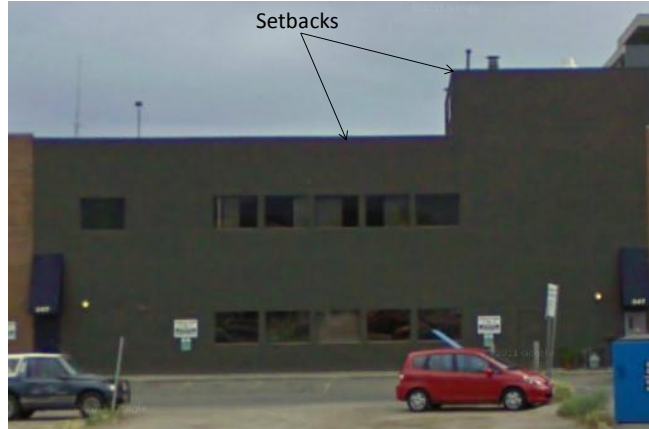
Figure 2-9: Example of vertical irregularities in Kelowna city, Canada
