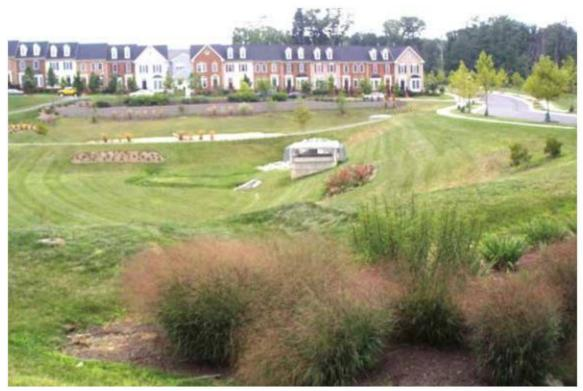
Figure 10 Example of a Dry Pond
