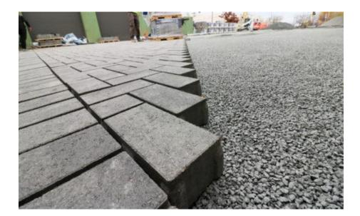
*Figure 4 Example of Partial Installation of Pervious Pavers* Source: Mississippi Watershed Management Organization
