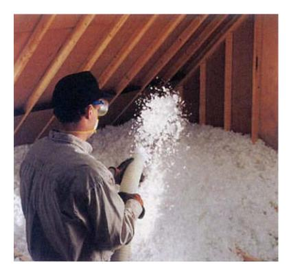
Figure 2 - Blown in Cellulose Insulation (Green Solutions Magazine, 2008)
