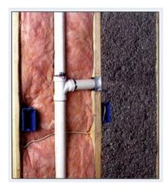
Figure 4 - Fibreglass (L) and Cellulose (R) Insulation (Houle Insulation Inc., 2009)
