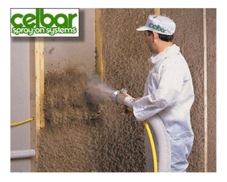
Figure 3 - Sprayed Cellulose Insulation (Celebar International Cellulose, 2010)
