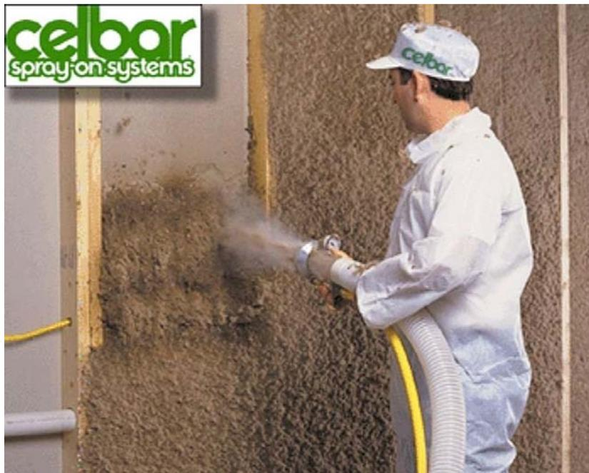
Figure 3 - Sprayed Cellulose Insulation
